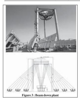
Managed by Masdar Institute, the Beam Down Plant has the potential to convert sunlight into electricity in a more efficient, lower-cost way than other technologies. By placing the receiver at the base of the tower (ground level), the thesis is that it will eliminate the energy loss resulting from pumping the fluid to an elevated receiver.
